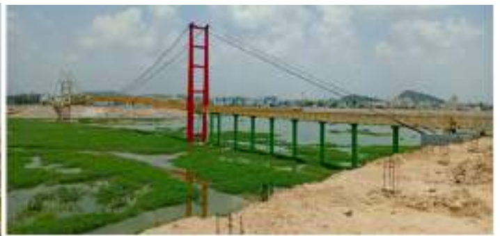
Cable Bridge at Mahabubnagar
