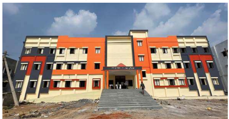
TGEWIDC - Construction of Dormitory Block in Nizamabad
