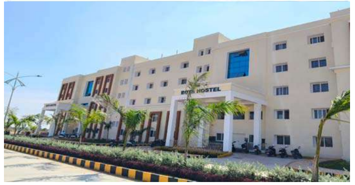
TGMSIDC - Construction of Boys Hostel to Medical College in Nalgonda
