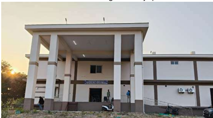
Construction of Central Medicine Store - Bhadradi Kothagudem
