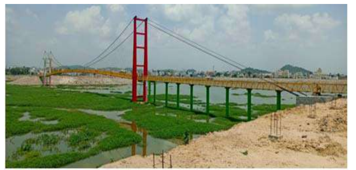
Cable Bridge at Mahabubnagar
