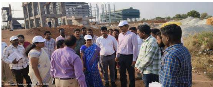
TPQC Inspection of TGOILFED works
